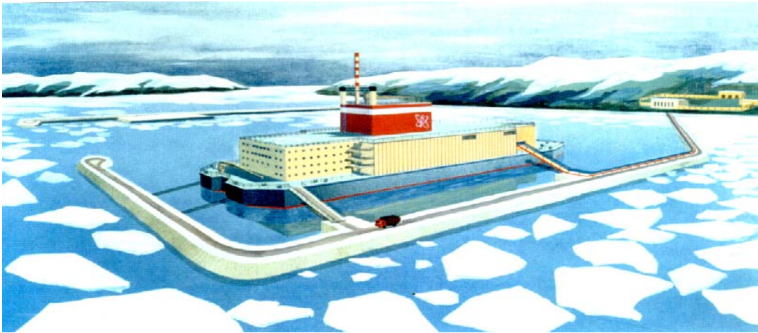
Pic.4. A FNPP attached to its protective mooring.
